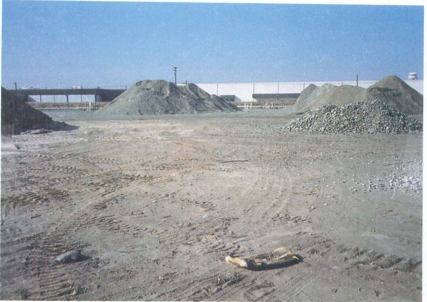
SITE 22 - LOOKING WEST
