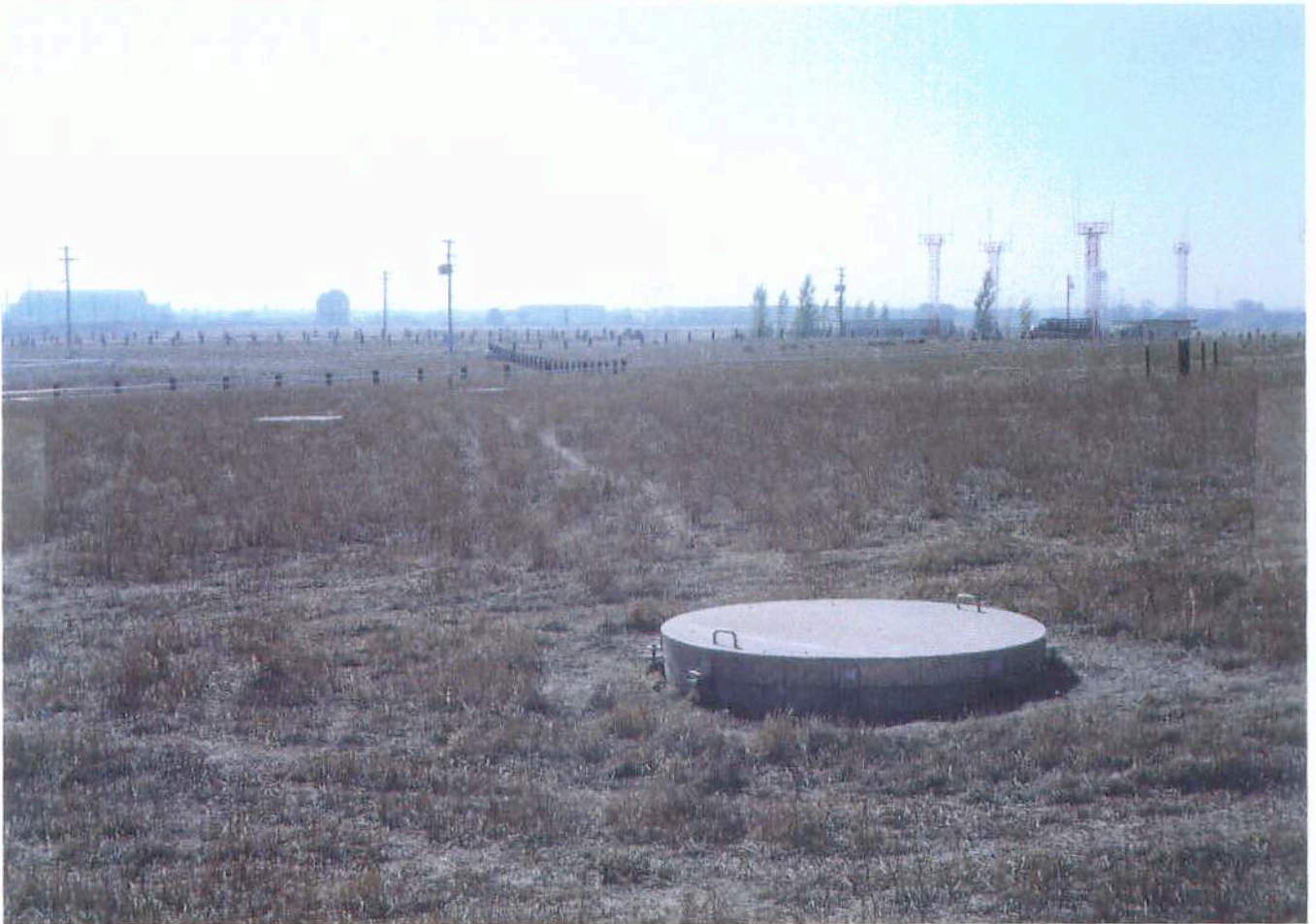
SITE S AND T - LOOKING SOUTH
