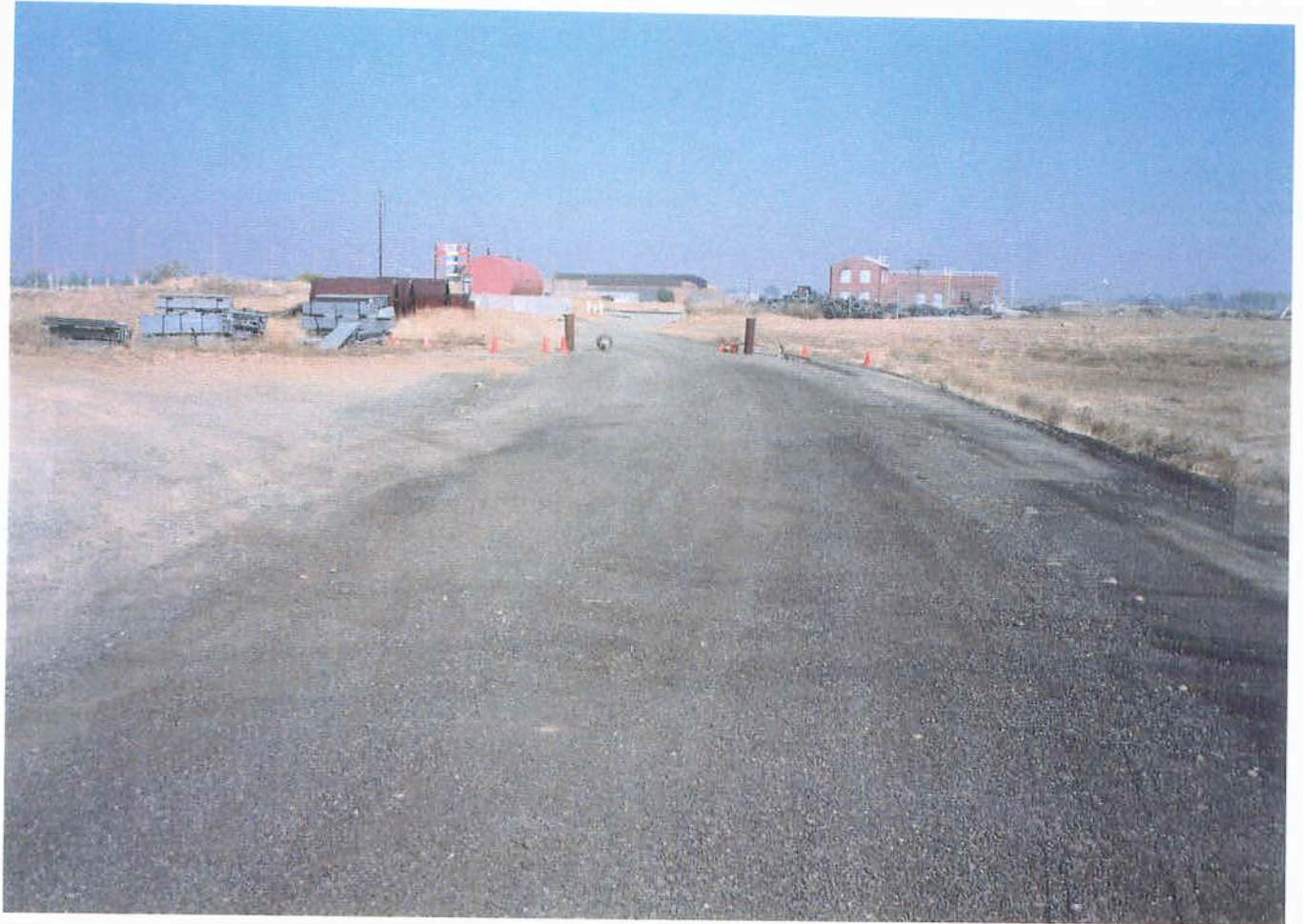
SITE 13 - LOOKING NORTH
