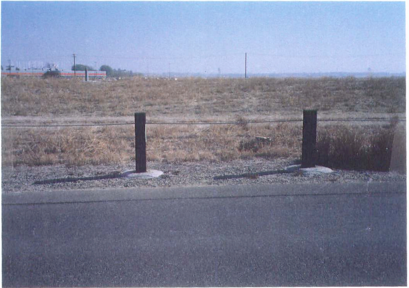
SITE 2 - LOOKING EAST
