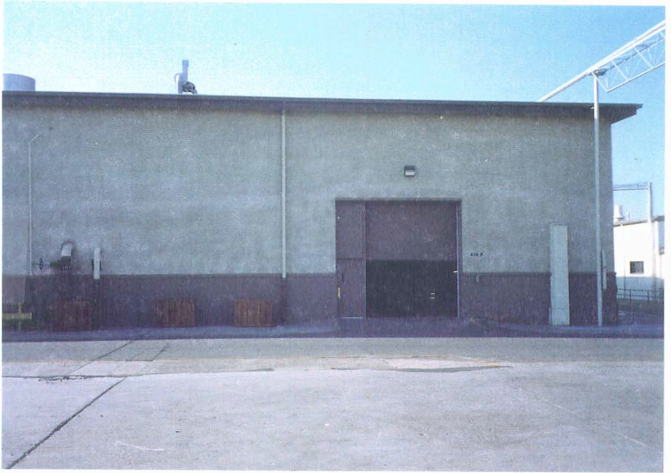
SITE 38 - LOOKING WEST
