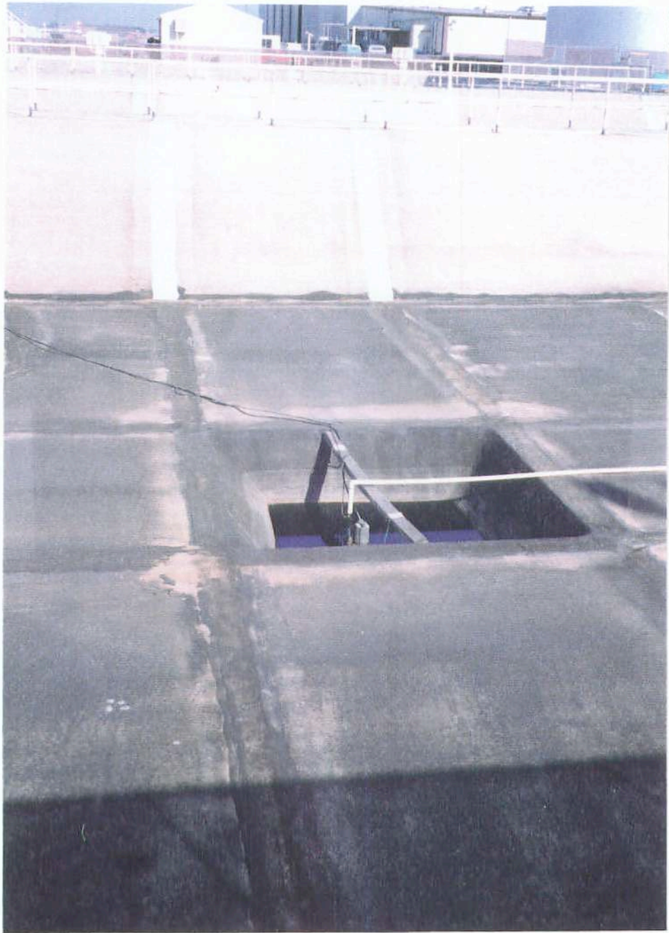
SITE 42 - LOOKING NORTH
