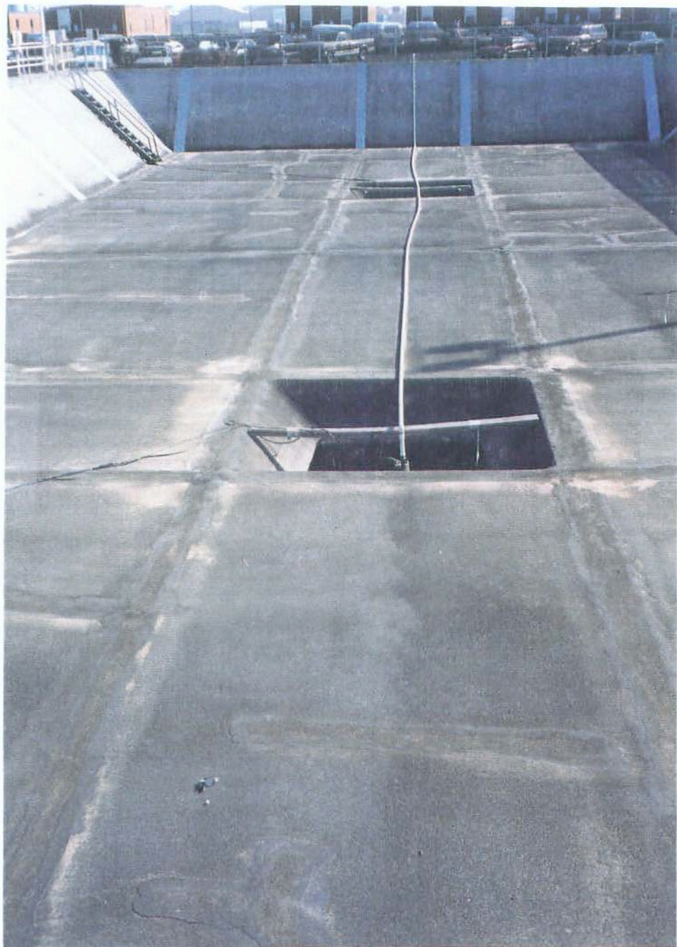
SITE 42 - LOOKING EAST
